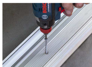
Sliding door track installation
